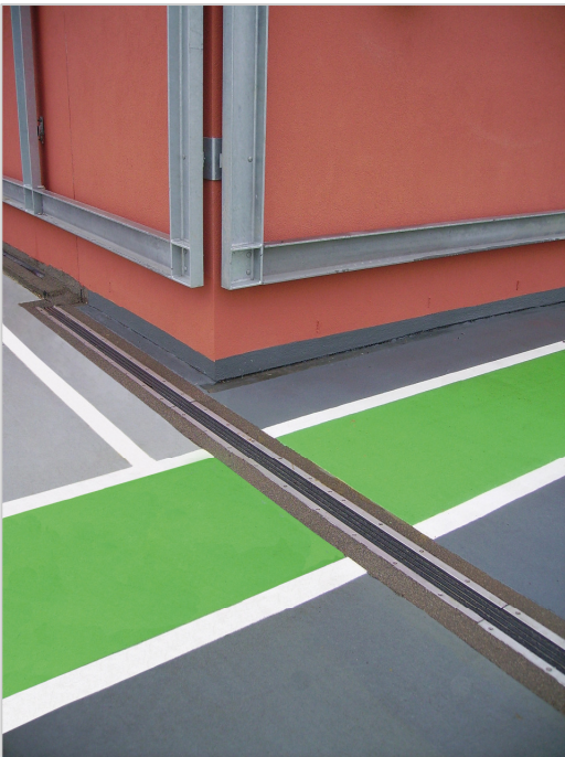
Figure 1: The UCP joint by USL StructureCare is designed to interact completely with waterproofing systems such as Conideck.
